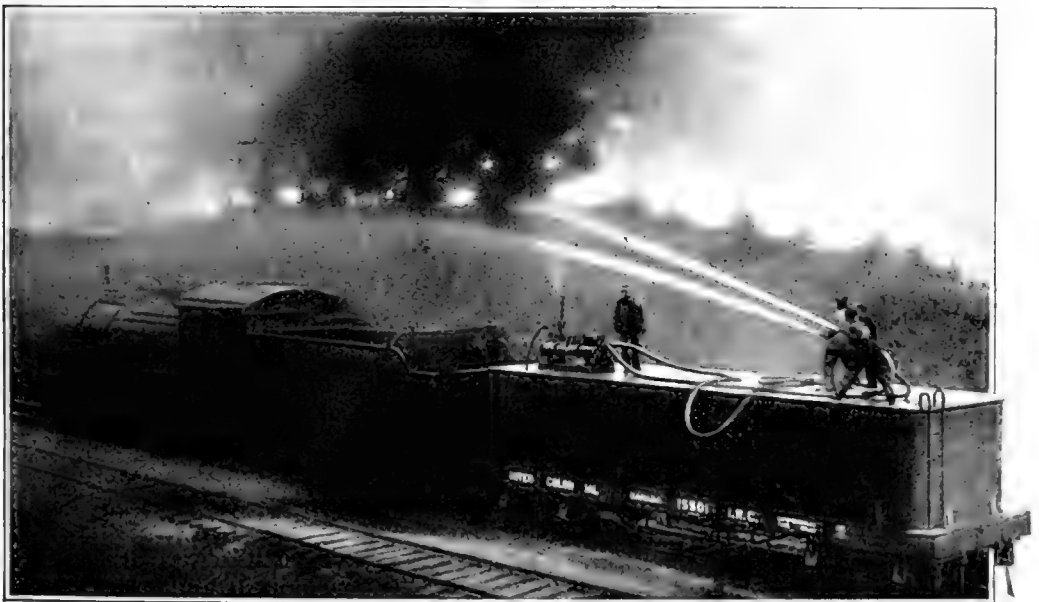
The fire-fighting apparatus is kept under steam so that it can be quickly transferred to any point on the railroad's system where fire may be threatening property worth millions
